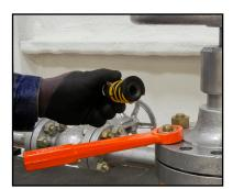
Remove the HAMMERTIGHT wrench retainer.
