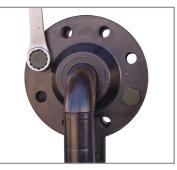
If necessary, use a second tool and turn until the bolt holes are in alignment and insert flange bolts.
